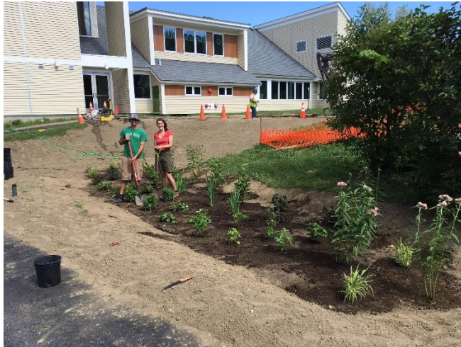
A rain garden built at Warren School, supported by Friends of the Mad River. Image credit: Friends of the Mad River
